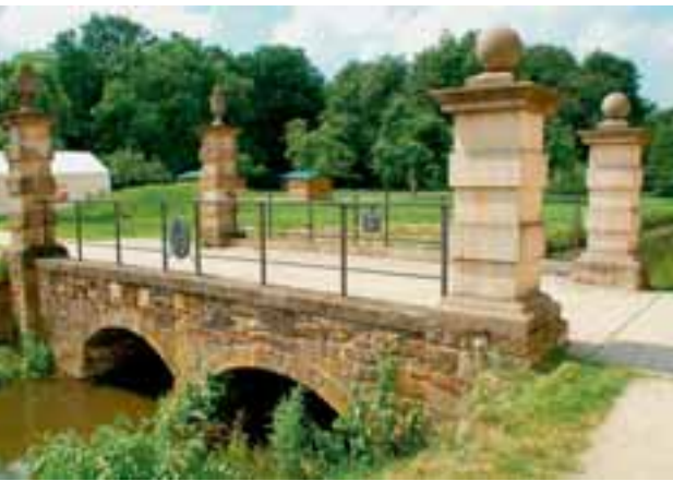
Parkbrücke in Gravenhorst
